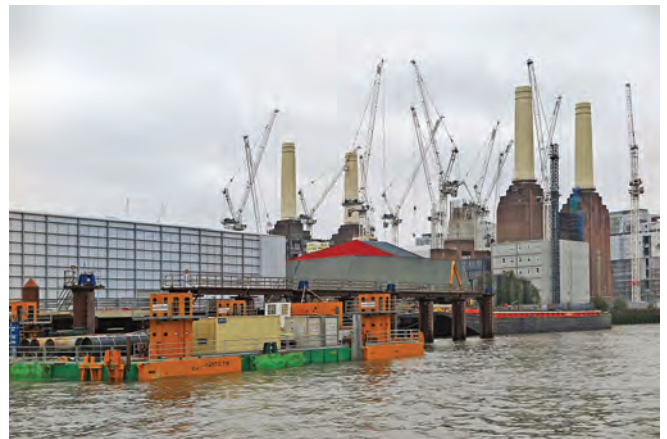
Main tunnel drive site at Kirtling Street, Battersea
